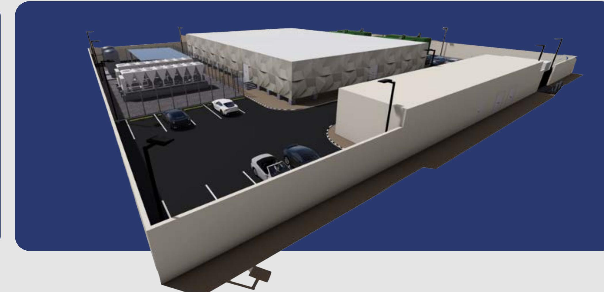
Prefabricated AI data centers are modular solutions designed to support AI-driven workloads efficiently and sustainably. These centers are built off-site and delivered as ready-to-deploy units, offering several advantages over traditional data centers.
